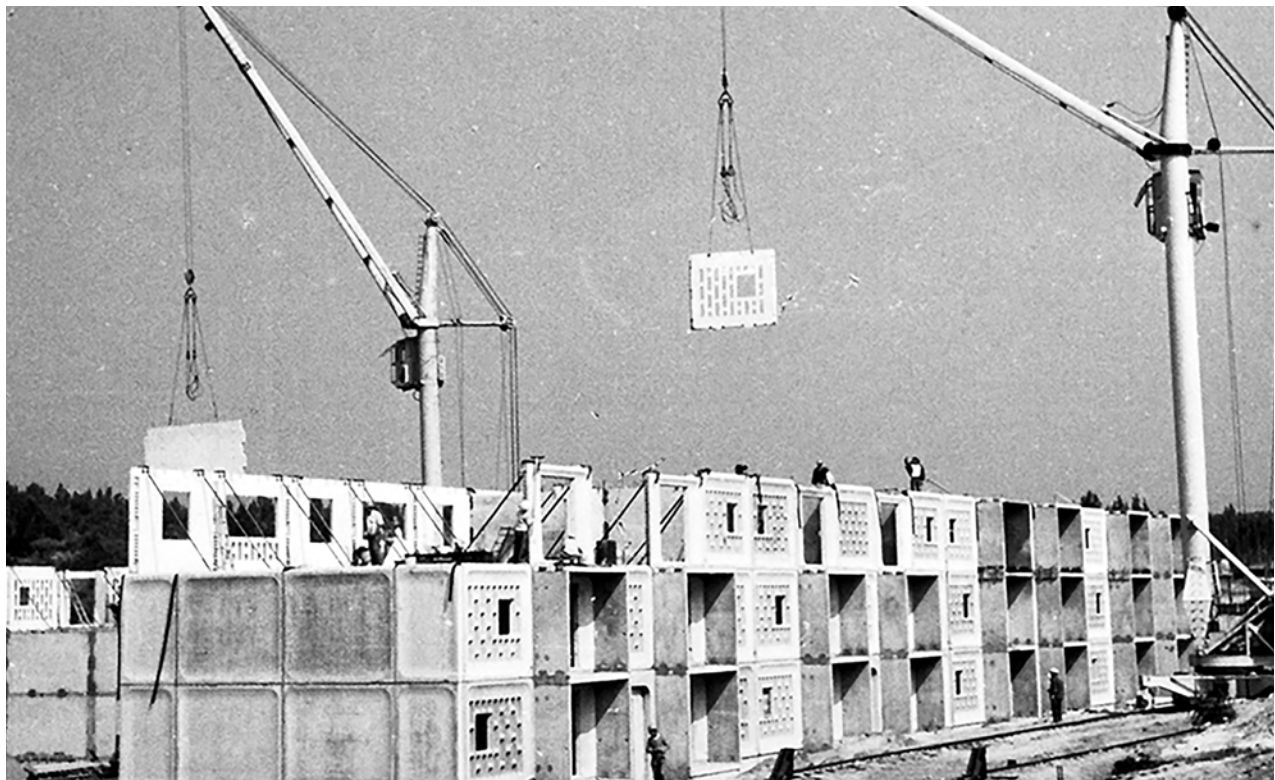
Image 94: Construction using KPD panels
