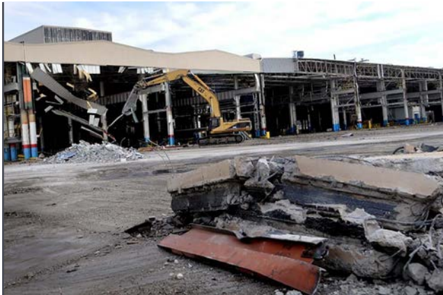
2011-2012 The building is demolished.
