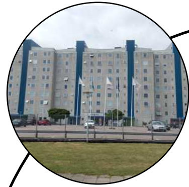
Re-use of Existing Infrastructure Rosengard, Malmö Sweden
