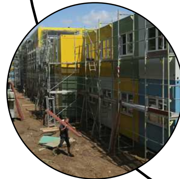
Re-use of Existing Objects Shipping Containers, Germany
