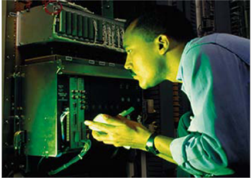
HVACR technicians repair heating, cooling, and refrigeration systems.
