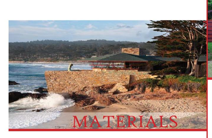
The material choices for the Walker Residence were a very important part of the designing the building to fit into the site. The house rises out of the sand on a stone foundation. The profile line of the porch suggests the feeling of a cliff to the viewer. Behind the porch, the three walls of glazing creates the illusion of the house receding from the beach. The low sloping, copper roof with deep overhangs grounds the building.
